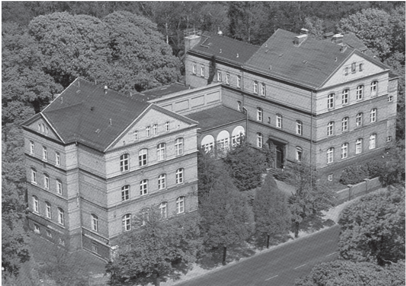
Fig. 5 Institute of forensic medicine at the Charité, formerly Humboldt-University Berlin. Built from 1884 to 1886, closed 2005
